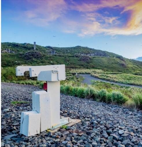
The water cannons are the heart of a robust defense strategy, which includes low-profile fire hydrants, fuel and firebreaks, and a concrete road to support firetrucks. The water cannons are strategically placed near vulnerable roosting/nesting trees where vegetation, terrain and winds would push fires.
